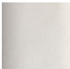
Plaster smooth finish
