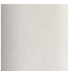
Plaster smooth finish
